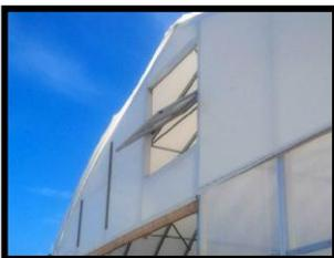
5. **OPENING REQUIREMENTS FOR FORCED OR NATURAL VENTILATION** (if required) need to be considered BEFORE starting to close an end. Fans and louvres will also limit your choices of doors.
