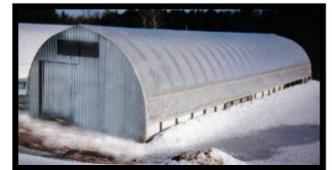
3. **COVERING TYPE** – in our packages the end covering is usually the same as the roof, either clear *plastic*, white *plastic* or woven *tarp*. These are very inexpensive but not as durable, especially when there is a lot of handling. We can also supply Lexan or Dyneglass where appearance, long life and light transmission are important. Plywood or sheet metal can be installed where appearance, long life and non-light transmission are important.
