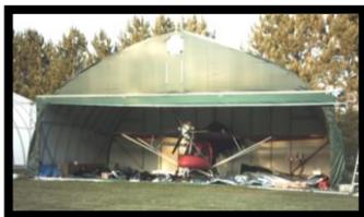
4. **ROLL-UP DOORS (soft cover)** should have two cross members attached to the *tarp* to prevent it from blowing inward. One is attached at the bottom and one in the middle. The middle one is attached to the cranking mechanism. There are also two verticals standing in front of your door posts with a space of 3" to prevent the door from billowing outward. **The of sealing the edges is the main issue with this system.**
