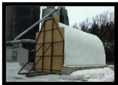
5. **END WALL REMOVAL** is an option if the intention is to seal up the building for the winter and then to have total access the remainder of the year. Installing an extra *wire insert* in the *wirelock channel* will allow simple removal of the end, while numbering the framing pieces will simplify the re-assembly.
