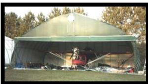
4. **ROLL-UP DOORS (soft cover)** should have two cross members attached to the *tarp* to prevent it from blowing inward. One is attached at the bottom and one in the middle. The middle one is attached to the cranking mechanism. There are also two verticals standing in front of your door posts with a space of 3" to prevent the door from billowing outward. **The of sealing the edges is the main issue with this system.**
