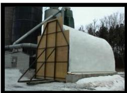
5. **END WALL REMOVAL** is an option if the intention is to seal up the building for the winter and then to have total access the remainder of the year. Installing an extra *wire insert* in the *wirelock channel* will allow simple removal of the end, while numbering the framing pieces will simplify the re-assembly.
