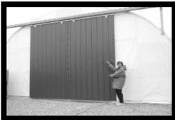
2. **SLIDING DOORS** should be 1"-2" bigger than the opening to allow for sealing. The track should be fastened to the side of the header and be 50% longer than the width of the door. If the track extends more than 2' past the curve of the building, the end should be supported. **It is usually desirable to slide a double door in one direction rather than splitting it because sealing the middle against drafts is very difficult.**
