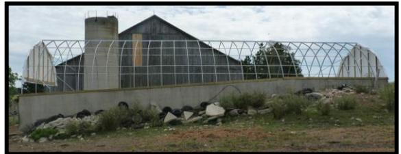
When significant excavation has been done, **the anchoring system MUST be set into concrete.**
