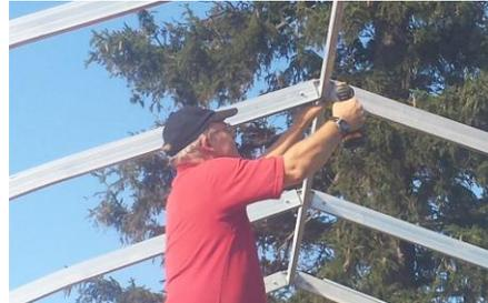
Tape any connections with duct tape to ensure nothing will rub on the cover
