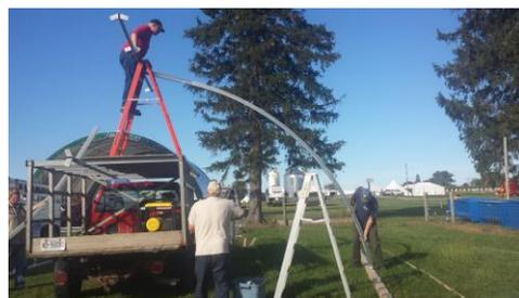
Flip the arch right side up slide it into the **middle** ridge stub, and over the base bracket or anchor post
