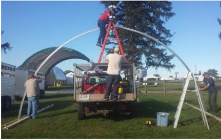
get **one pair** of arches standing attached to the middle ridge stubs before continuing
