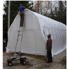
**General Notes:** The curved part of the *hoop* is usually the bottom; the straight part is the top. For structures that have been supplied as a cathedral unit (for RV, boats, etc.) the curved part goes up and the long straight part goes down.
