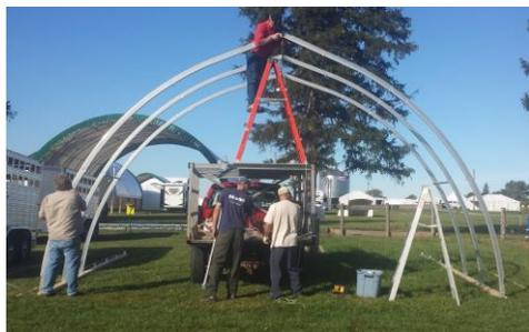
make sure you are securing each arch to the ridge stub before continuing, then secure the two sections of ridge together
