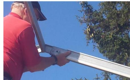
slide the arch into the ridge stub
