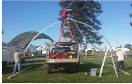
continue with the next pairs in the same manner fastening the arch to the ridge and the base bracket until all stubs in the ridge have been used
