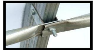
Repeat this process for each diagonal line of *purlins* in all four corners. **Unless your building is PERFECTLY level with the *hoops* PERFECTLY square, the *braces* will look different at the two ends (this is acceptable).** If your building has 2' *hoop* spacing, you will be attaching to alternate *hoops*... i.e., cross over and attach to the next *hoop*.
