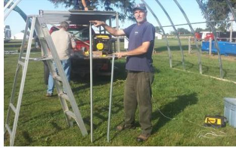
The holes drilled in each end are spaced at the same spacing as the *hoop* spacing. The tabs with the holes of 2 *purlins* overlap and are bolted to the underside of the *hoop* (structure).
