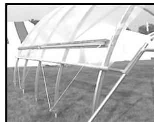
4- Thread the braided rope which is supplied, continuously through all the eyebolts. This rope holds the pipe against the building during windy conditions. It is usually tightened somewhat during the winter.
