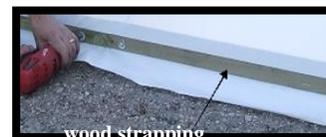
4- If you are **using wirelock along the sides, start from the middle and work toward the ends.**
