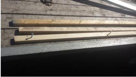
ensure the screws are in the 1x2 to prepare for fastening the cover to the base
