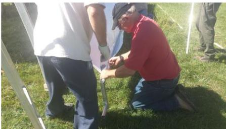
roll the cover around the roll up pipe strap
