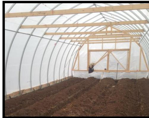
This **interior view** of a moveable structure shows how the bottom of each end must have some sort of flap so that when moving over a crop or off the crop you will not disturb the plants that are there. The interior horizontal lumber is to supply support for a crop of tomatoes.
