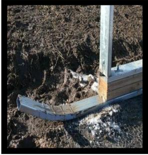
A variation on the base is to put some wood between the 2 layers of the base rail. The advantage of this is that you get some extra height to work with for fastening the
