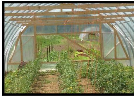
It is very important that you have adequate ventilation on your moveable structure. End to end ventilation will only work on a short structure that is facing into the wind.
