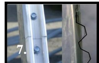
**Wirelock Insert:** the "zip-zag" stainless, heat-treated steel wire used in the wirelock channel to hold the covering in place (see photo 7, right)
