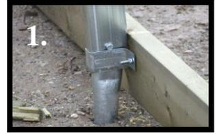
**Base Bracket:** is a formed strip of steel that uses lag bolts to secure it to the base beam. The hoop slides over top for fastening and stability. (see photo 2)
