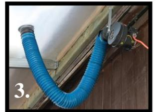
**Inflator Fan:** small fan that blows continuously to maintain an air space between two layers of plastic (see photo 3)
