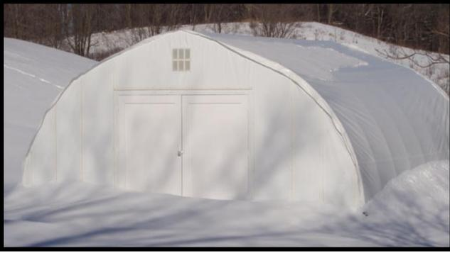
Our structures are designed in Canada with a *gothic* shape with a slippery cover to be lightweight and snow resistant. This encourages the snow to slide off quickly. **However! This is not an industrial high snow load building.** We do our best to always point out applications where the capacity of the structure is being compromised. Extra *hoops* are an economical way to increase wind and snow load capacity.
